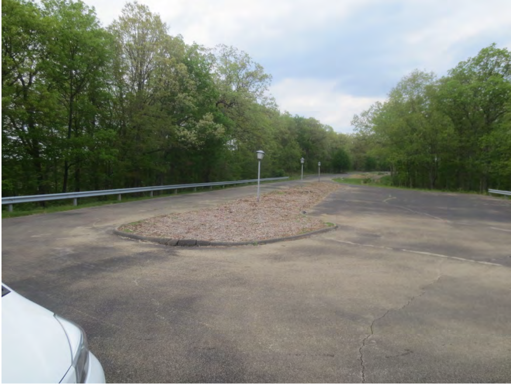
Parking lot north of Eagle's Landing building
