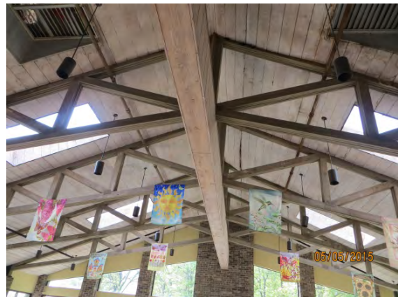
Figure 36 – Indoor swimming pool – pendant incandescent fixtures
