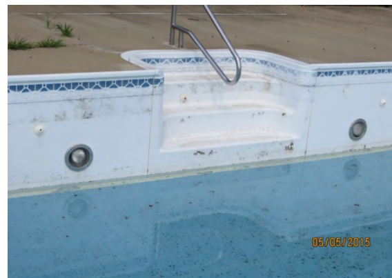
Figure 56 - Swimming Pool – Recessed with Gasket Fixture
