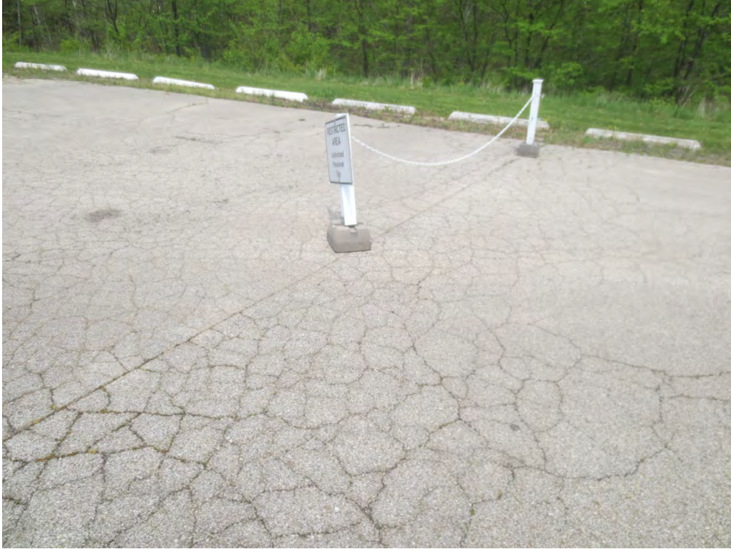
Wheel stops on north east side of lot located in grass
