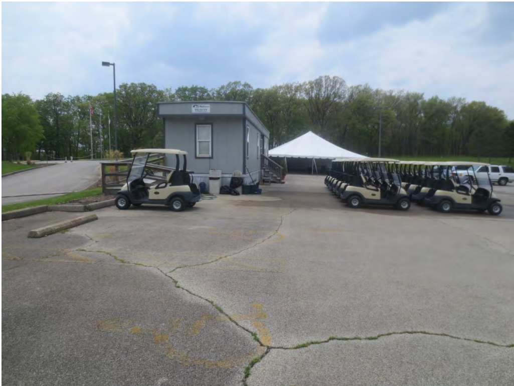
Golf cart parking / temporary Pro Shop trailer and tent
