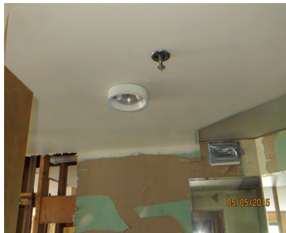
Figure 46 - Typical Bathroom Ceiling
