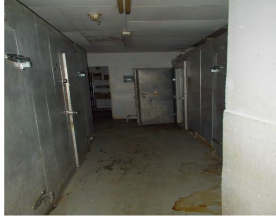
Figure 28 – Kitchen freezer lighting
