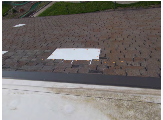
Figure 26 – Roof Patching
