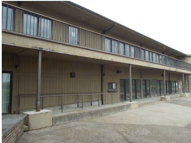
Note Exterior Ramp
