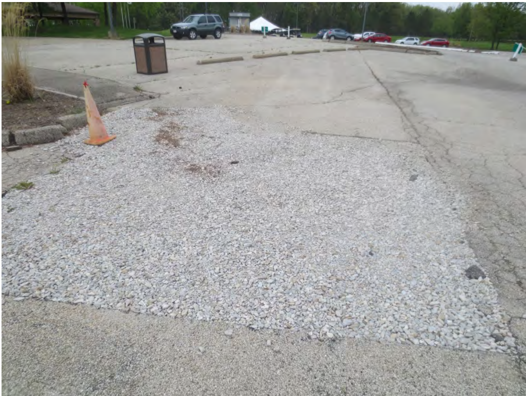
Approximately 15' x 15' area of gravel near loading dock
