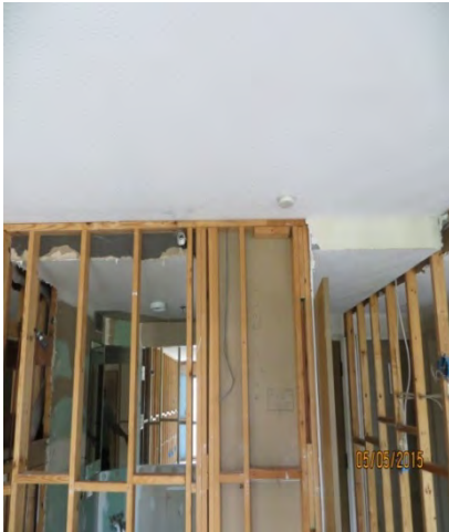
Figure 69 - Typical Smoke Detector in Guestroom
