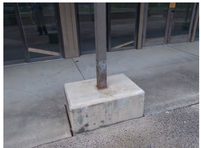
Figure 14 – Raised Pier and Steel Support
