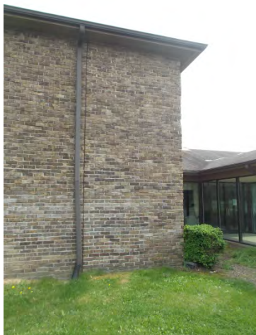
Figure 5 – Downspout
