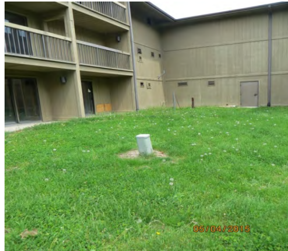
Figure 59 - Existing Telephone Service
