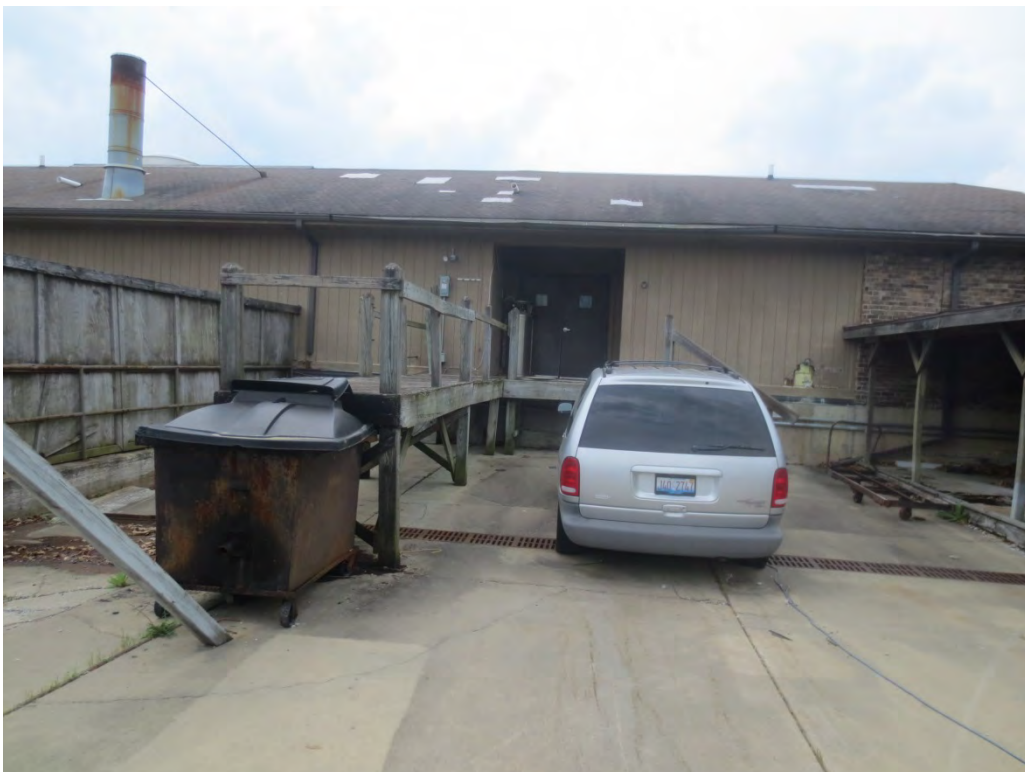
Loading dock area; note wooden dock platform
