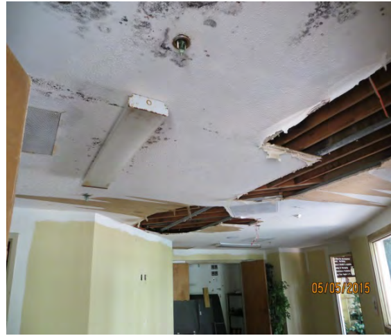
Figure 40 – Exercise room lighting
