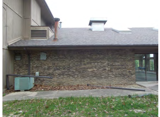
Figure 16 – Hotel Entrance Wall
