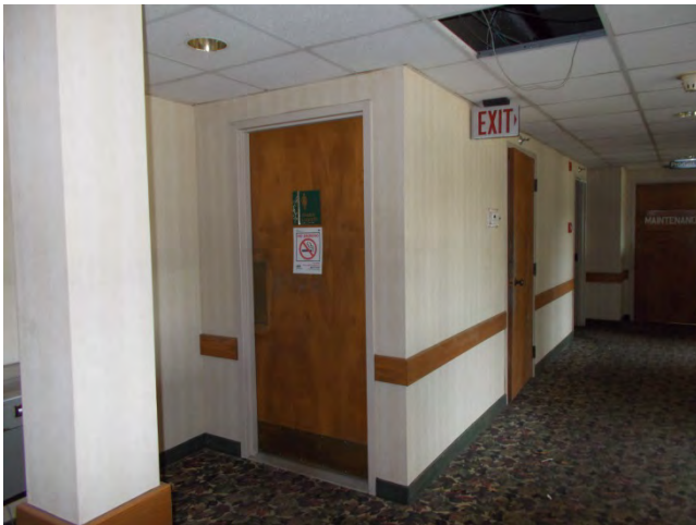
Toilet Room Access
