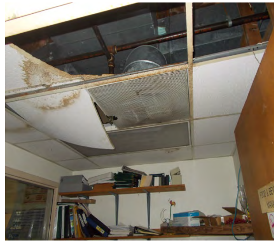
Figure 30 – Kitchen office lighting
