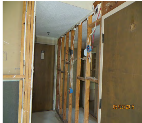
Figure 44 - Typical Suite Foyer
