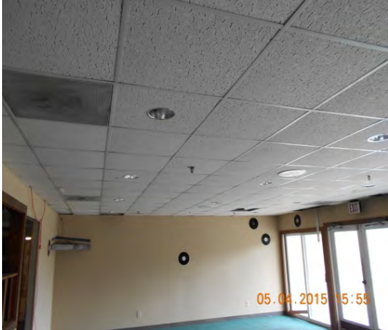
Figure 33 – Meeting room lighting
