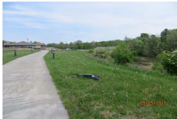
Figure 54 - Bollard Fixture Rooted-up
