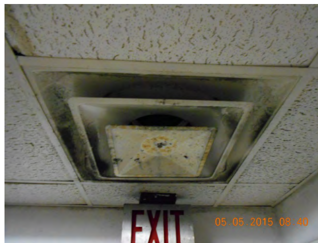
Figure 11 – Supply diffuser mold
