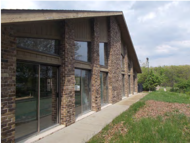
Figure 35 – Indoor Pool Building
