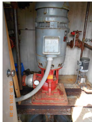
Figure 2 – Fire pump
