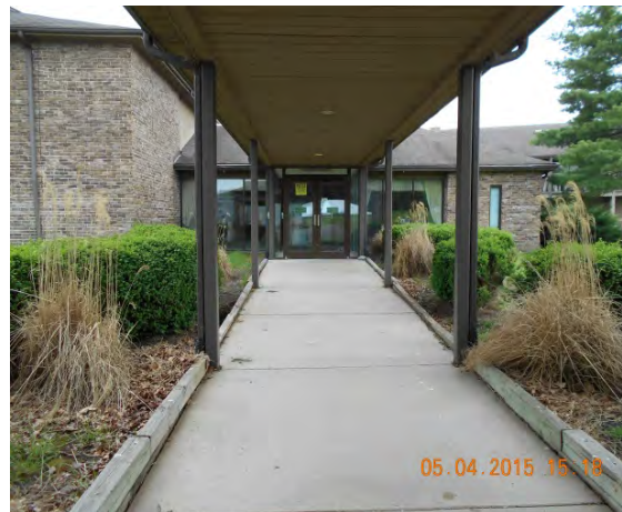
Figure 20 – Entry canopy to main lobby
