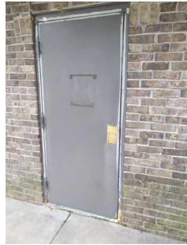
Figure 38 – Hollow-Metal Door without Hardware
