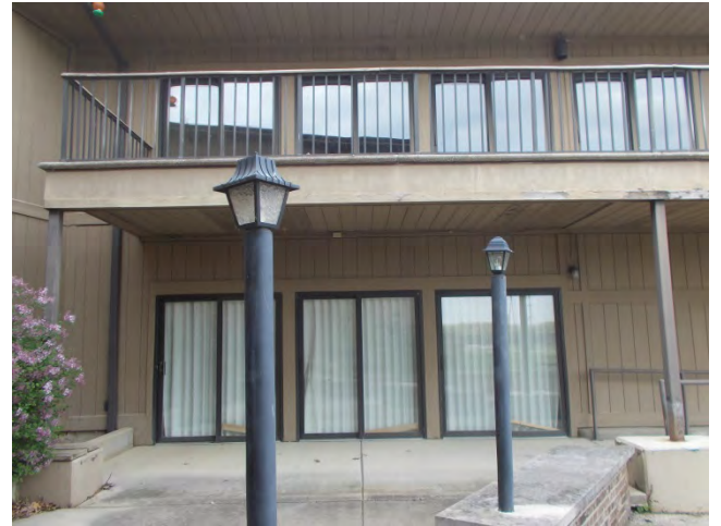
Figure 36 – Sliding Glass Doors
