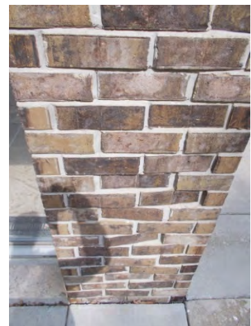
Figure 3 – Typical Pier Brick
