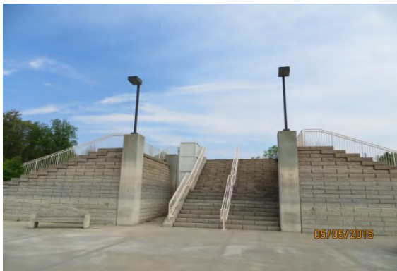
Figure 55 - Typical Boat Dock Lighting
