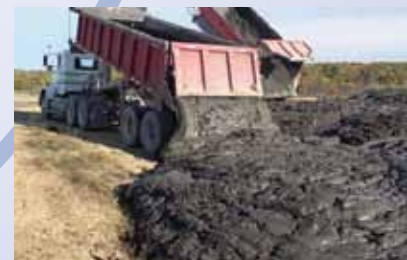
Sediment that the day before was on the bottom of the lake is placed on the clay liner of the Pekin Landfill to provide soil for final vegetative cover.
