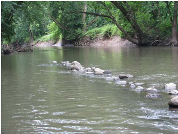
Figure 3. Instream Restoration Longitudinal Stone Habitat Structure
