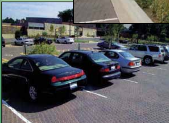
Morton Arboretum parking lot in use... notice holes in pavement to allow rainwater and snow to filter into the gravel base instead of running off into the lake and river.
