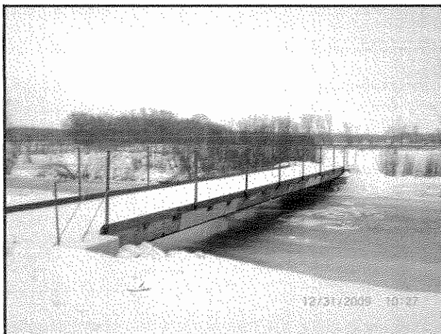
Railcar Handrail Installation Looking South
