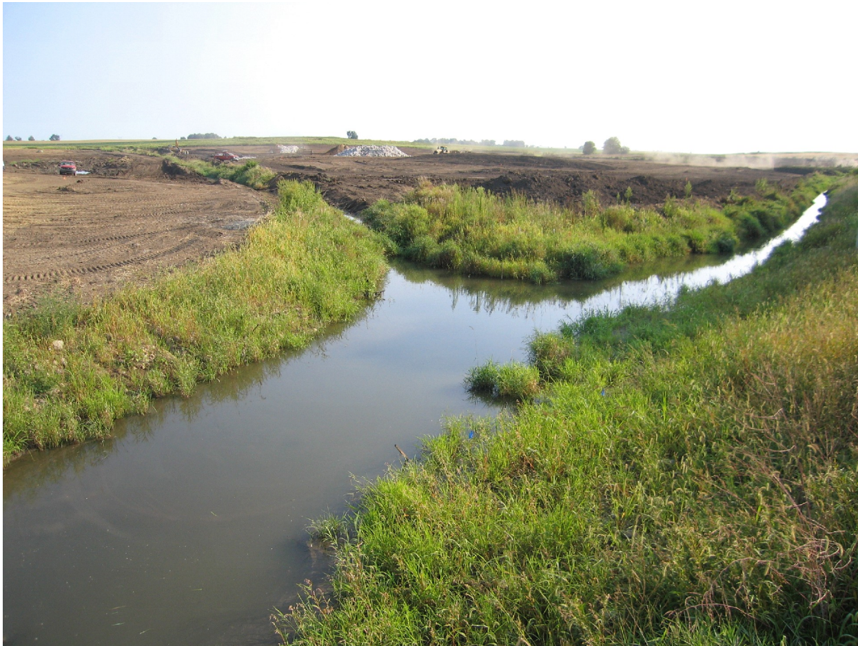
Figure 19. Lowering the floodplain to re-establish a natural flood regime and create wetland habitat within the Phase 1 reach of the restoration project.
