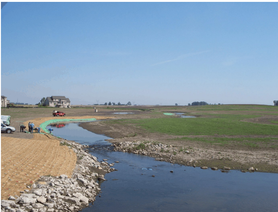
Figure 18. The project area was seeded under the direction of Bryan Cross of Kaskaskia Engineering, and the stream banks were blanketed for protection against erosion.
