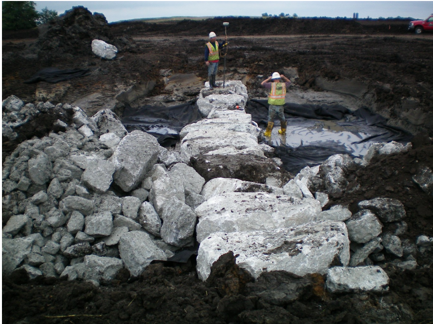
Figure 13. The peak stones set the height of the Newbury weirs. This was checked carefully with GPS equipment, as riffle height is critical to the function of the weir.
