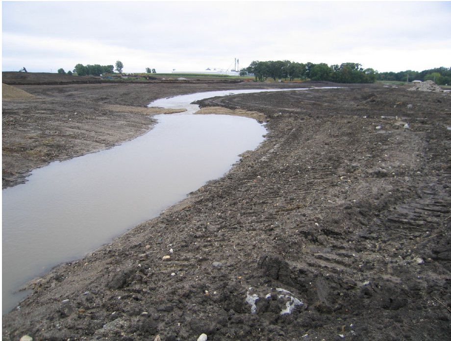
Figure 15. This view shows the newly constructed channel immediately following introduction of stream flow. The rip rap placed in the outside bends has been covered with soil to allow the establishment of vegetation. The water is in its initial stages of carving its path through the CA6 mix over Newbury weir.
