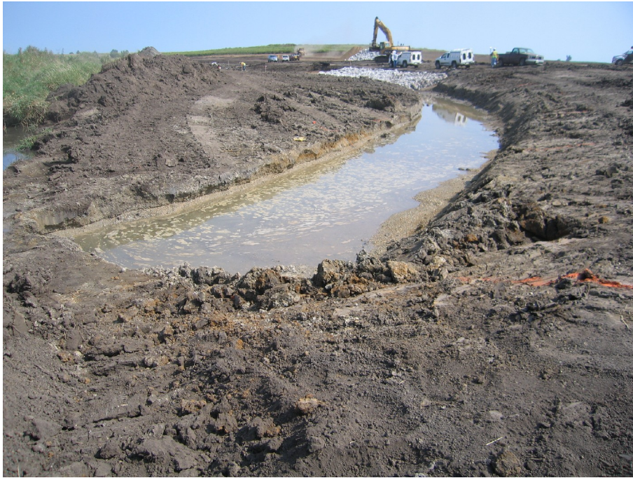
Figure 9. The new channel was constructed “in-the-dry” adjacent to the existing channel (seen in the upper left hand corner of this photo). Water within the excavation is groundwater seepage, which is a contributing factor to the high quality of this stream system.
