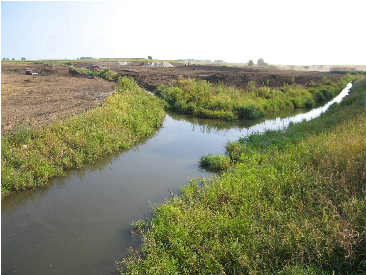
Figure 19. Lowering the floodplain to re-establish a natural flood regime and create wetland habitat within the Phase 1 reach of the restoration project.
