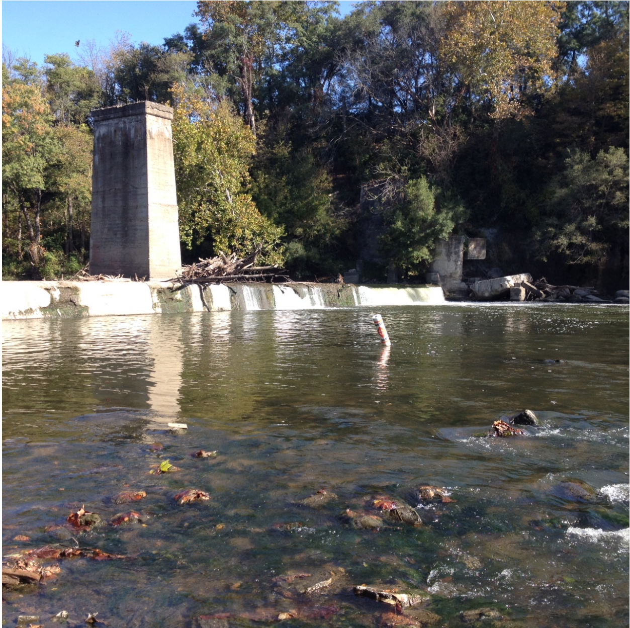
Figure 7 – Danville Dam photo from October 14, 2015 showing seepage along the face of the dam during low flow conditions.
