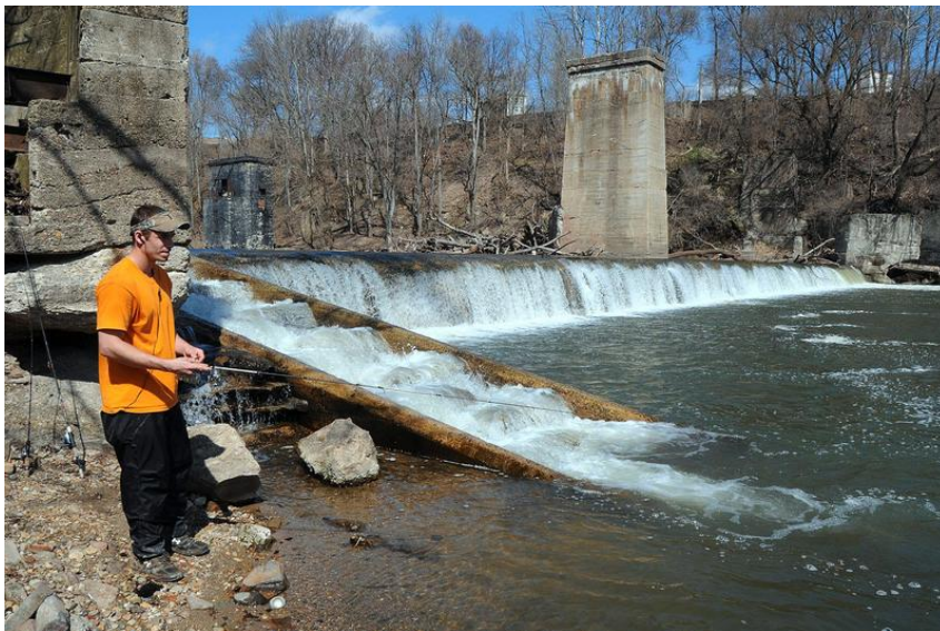
Figure 6 – Danville Dam during above normal flow conditions, fish ladder in foreground.
