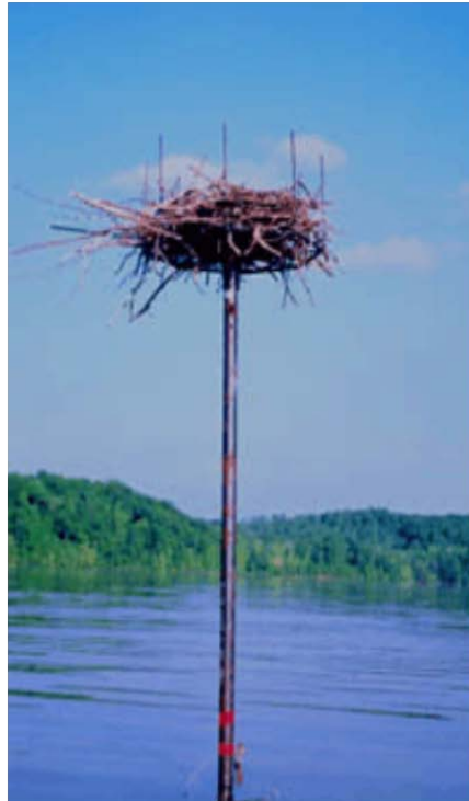
Figure 3. An osprey nesting platform. Note the desirable features of (1) robust, durable construction, (2) protection from mammalian predators, (3) elevation above surrounding features and unobstructed access for osprey to arrive and depart from the structure, (4) proximity to foraging areas, and (5) relative security from roadways, utility lines and other potential hazards.
