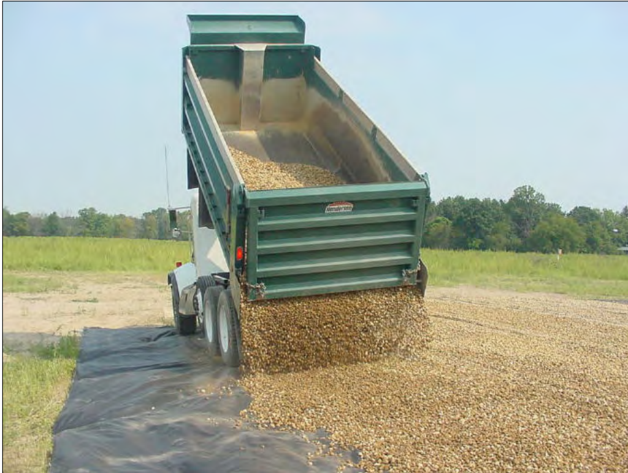
Spreading the rock.
