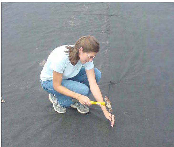
Pinning the fabric in place.
