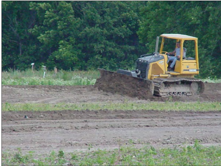
Constructing the island.
