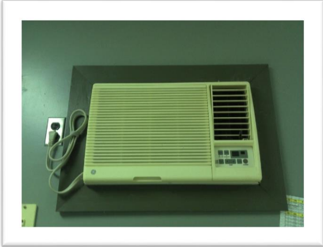
Old air conditioner, wall water damage, wasp nest
