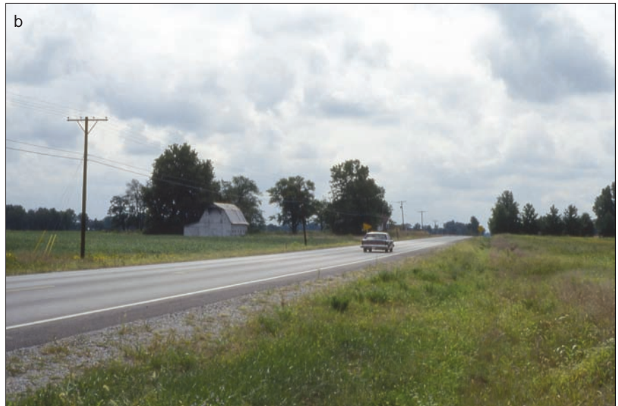
Figure 13 Examples of a road subsided (a) over a longwall panel and (b) repaired.
