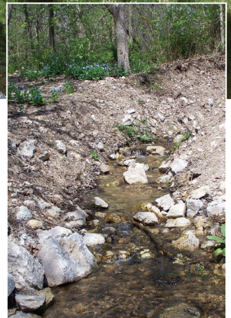
The bypass ramp was dug out to specified elevations (top), and then lined with rock (right).
