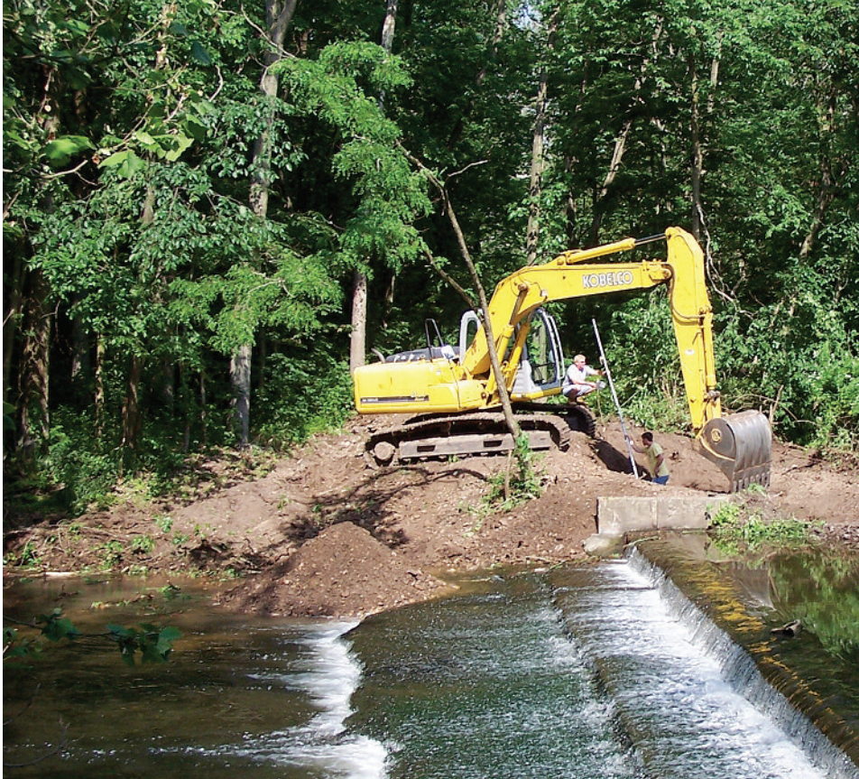
The bypass ramp was dug out to specified elevations (top), and then lined with rock (right).
