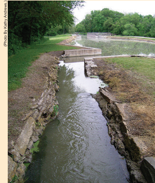
The Aux Sable spillway provides a visual clue of how water moved around the locks when gates were closed.
