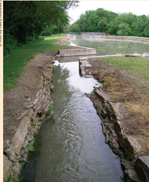
The Aux Sable spillway provides a visual clue of how water moved around the locks when gates were closed.
