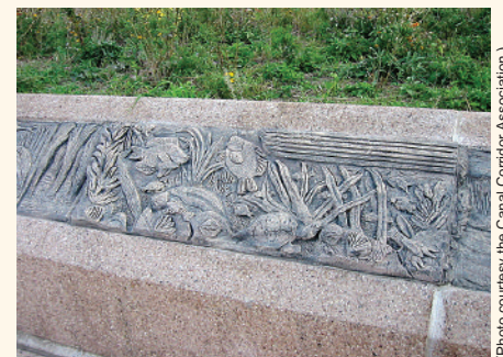
Railing at Canal Origins Park.
