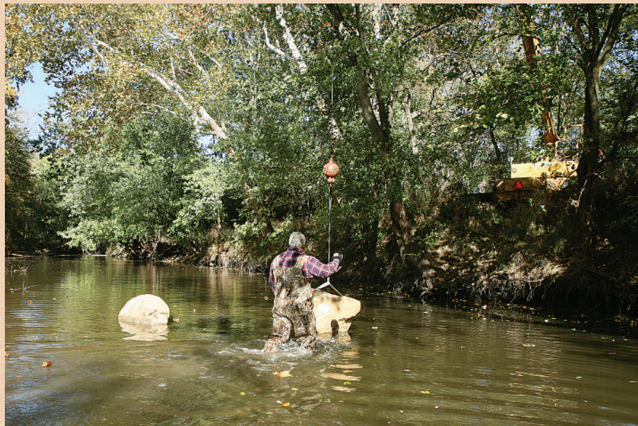
From the bank, a crane lowered boulders to a contractor for placement in the creek (below). A DNR biologist carries an armload of live mussels to be identified and moved prior to boulder placement (right).
