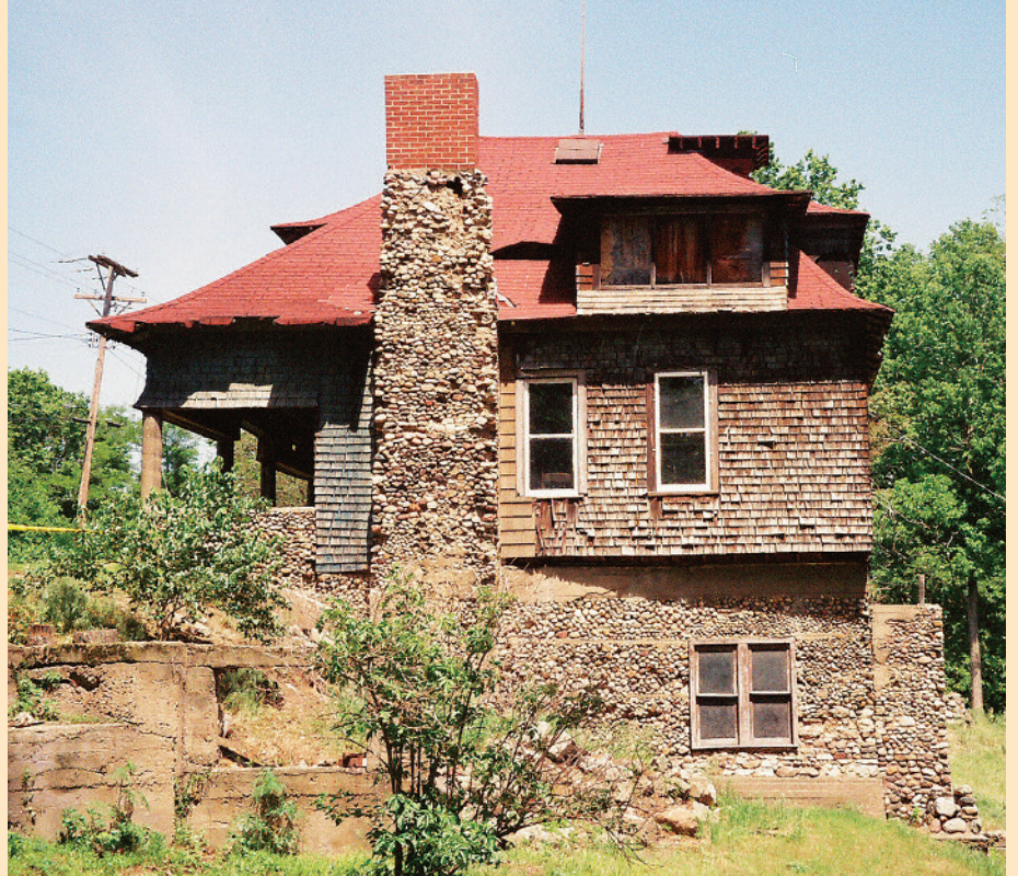
Charles Perdew used river rock for the foundation and chimney of his home built near the Illinois River in Henry.
