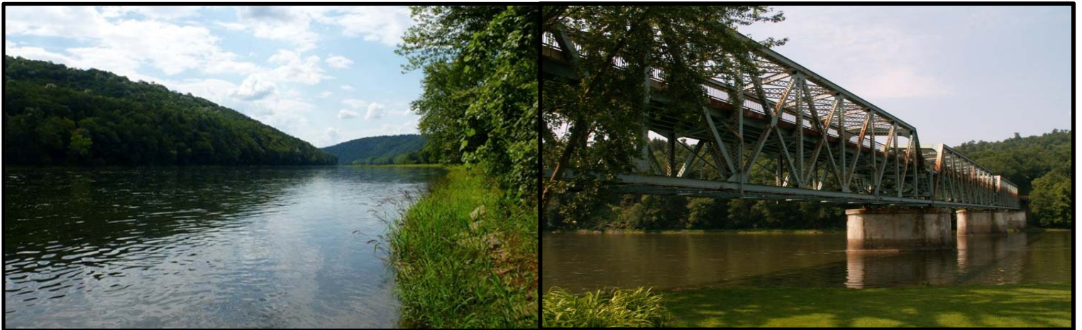
Figure 2. Pictures of the Pennsylvania bridge site along the Allegheny River (University of Illinois INHS presentation).
