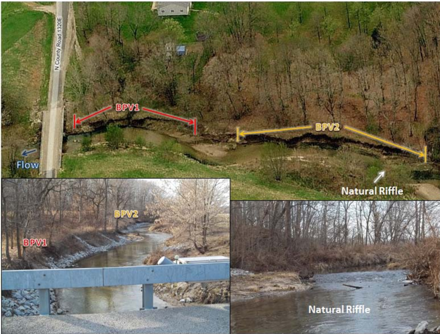
Figure 2. Condition of banks before peak stone installation at BPV1 and BPV2 (top-looking south) and after installation (bottom left-looking upstream). The single natural riffle in the restoration reach is shown in the bottom right (looking upstream) (natural riffle was undisturbed during construction).
