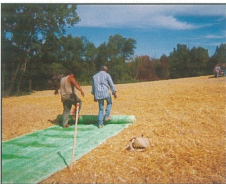
Above, a refuse pile in Grundy County. These piles usually contain shale, rock and some coal. Left, two workers apply an excelsior blanket to a reclamation site in Grundy County. The blanket contains mulch that protects soil from erosion and allows seeds beneath it to grow through the blanket.
