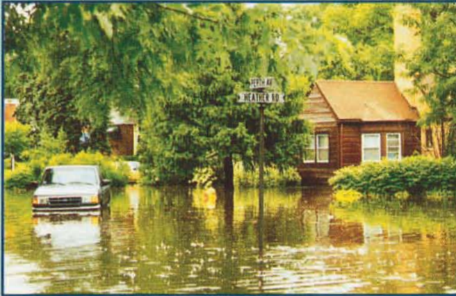
Flooding on Butterfield Creek
