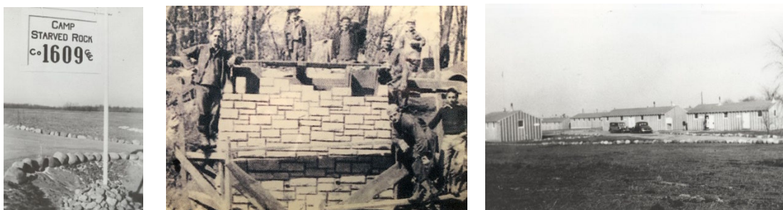
CCC men constructing LaSalle Canyon bridge.
