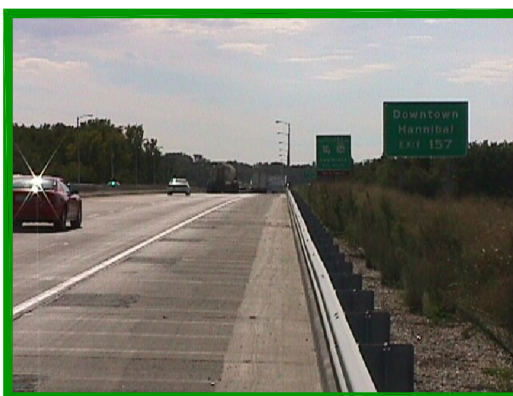
HANNIBAL BRIDGE CONNECTION
