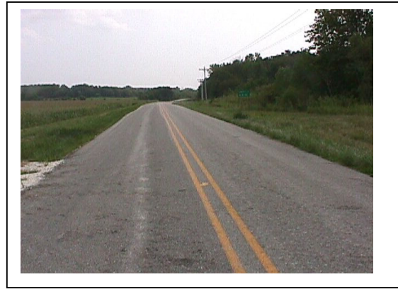
Figure 6-Typical County Road Shared Roadway
