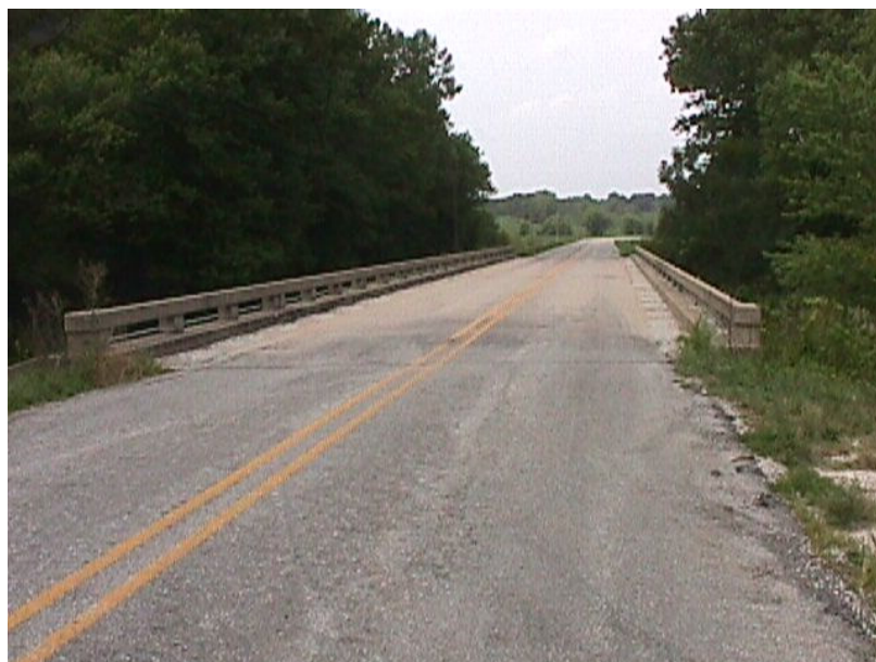
Figure 2- Bridge Over McKee Creek South of Siloam Springs
