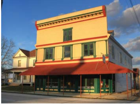
Connecting citizens and visitors through pedestrian and cyclist facilities and safe routes to cultural assets such as Center for American Archeology Visitors Center and Museum, often leverages more funding.
