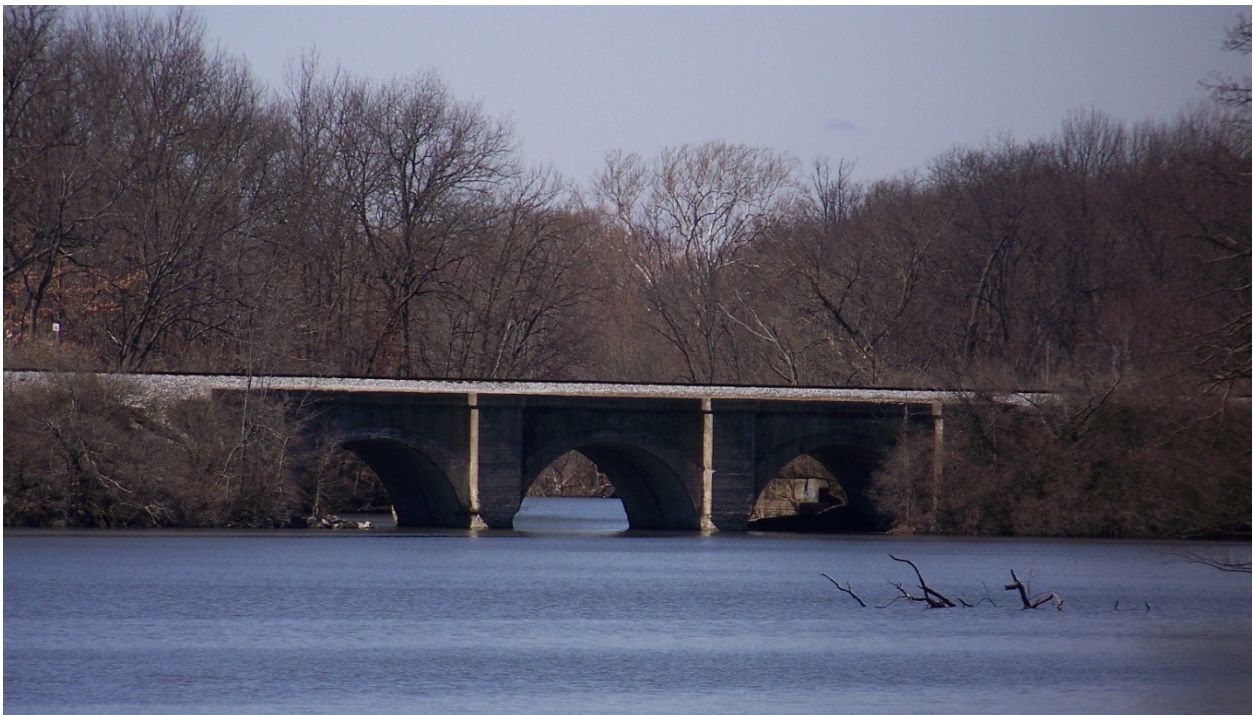
Railroad bridge over Twin Lakes
