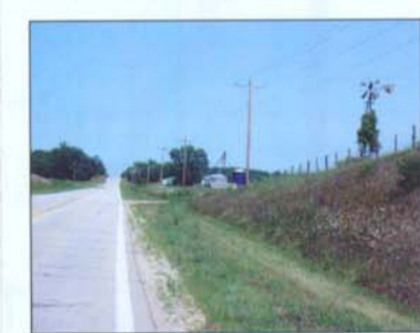
Road right-of-ways and shoulders can provide linear open space for future bikeways, signed sightseeing routes, snowmobiling, etc. Hoopole.
