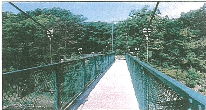
Rock Creek multi-use bridge, Kankakee River State Park Bike Trail
