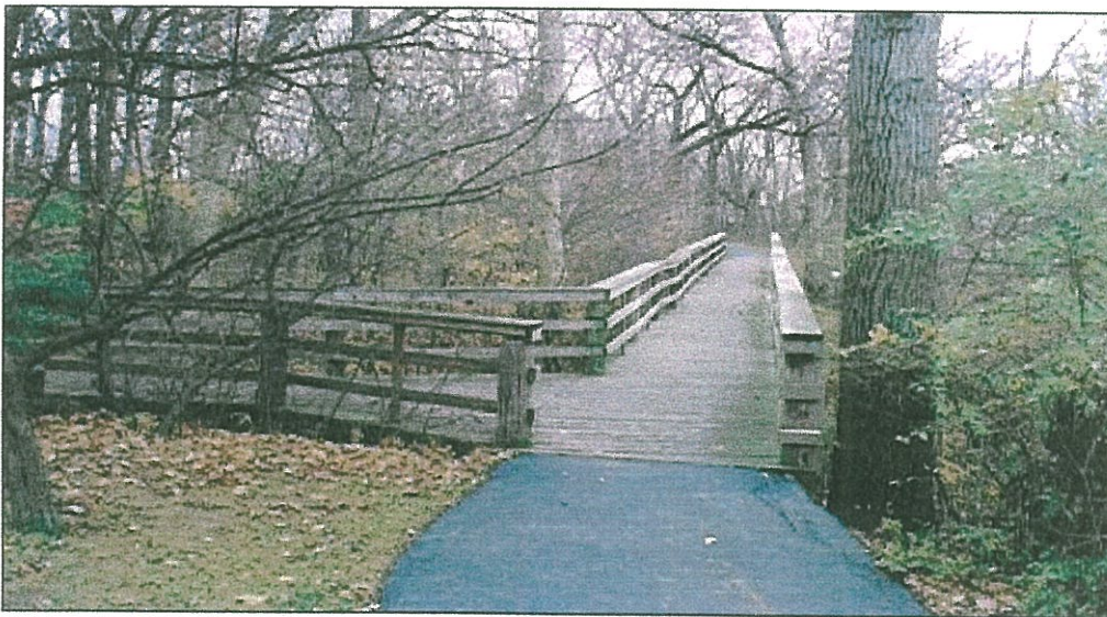
Example of an existing greenway, Briarcliff Estates, Bourbonnais, IL
