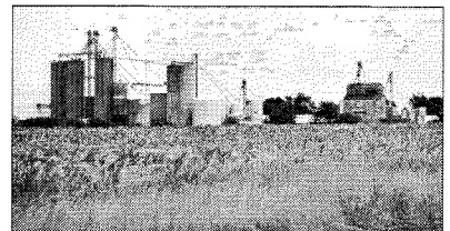
Old and New Elevators, Wing
