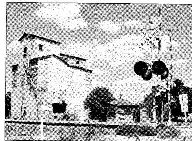
Abandoned Elevator, Cayuga
