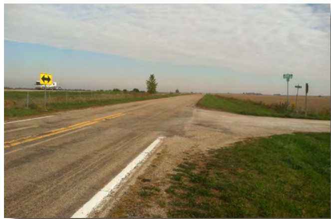
Trailway connection to Tazewell County | NE of Emden, IL
