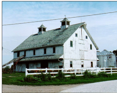
Barn near Pennington Point
