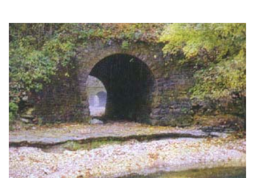
PEARL TWIN CULVERTS
