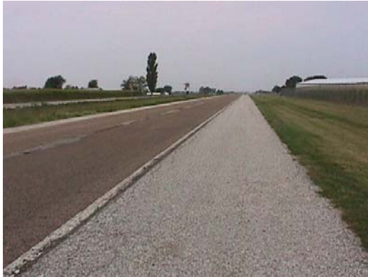
Figure 6 Typical Paved Shoulder on Highway Should Be Striped As a Bike Lane
