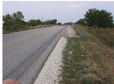
Figure 5 Example of Needed Paved Shoulder
