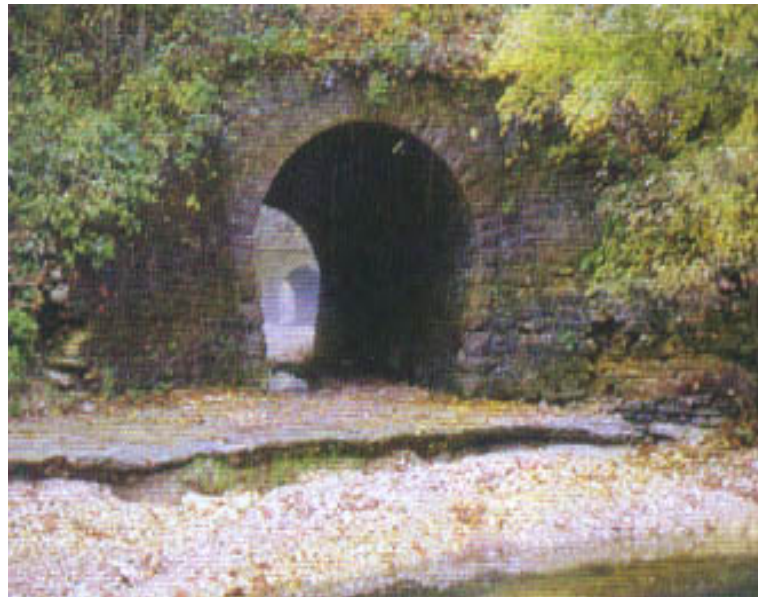
Figure 1 – Twin Culverts in Pearl
