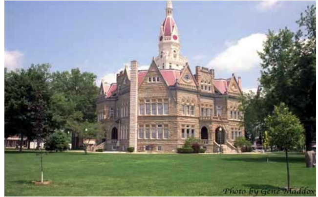
Figure 3 Historic Pike County Courthouse – Pittsfield
