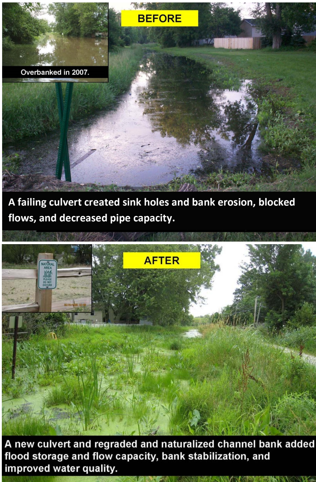
Figure 4.3: The Round Lake Drain ecosystem restoration project is an example of a flooding mitigation project in Lake County. Photos courtesy of Lake County Stormwater Management Commission.
