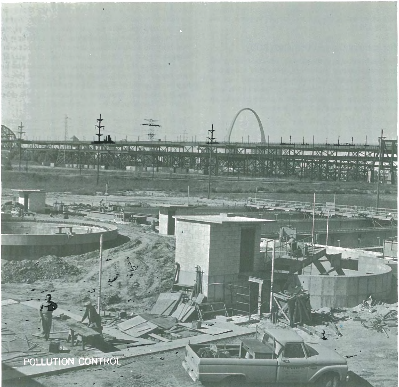
East St. Louis treatment plant under construction.
