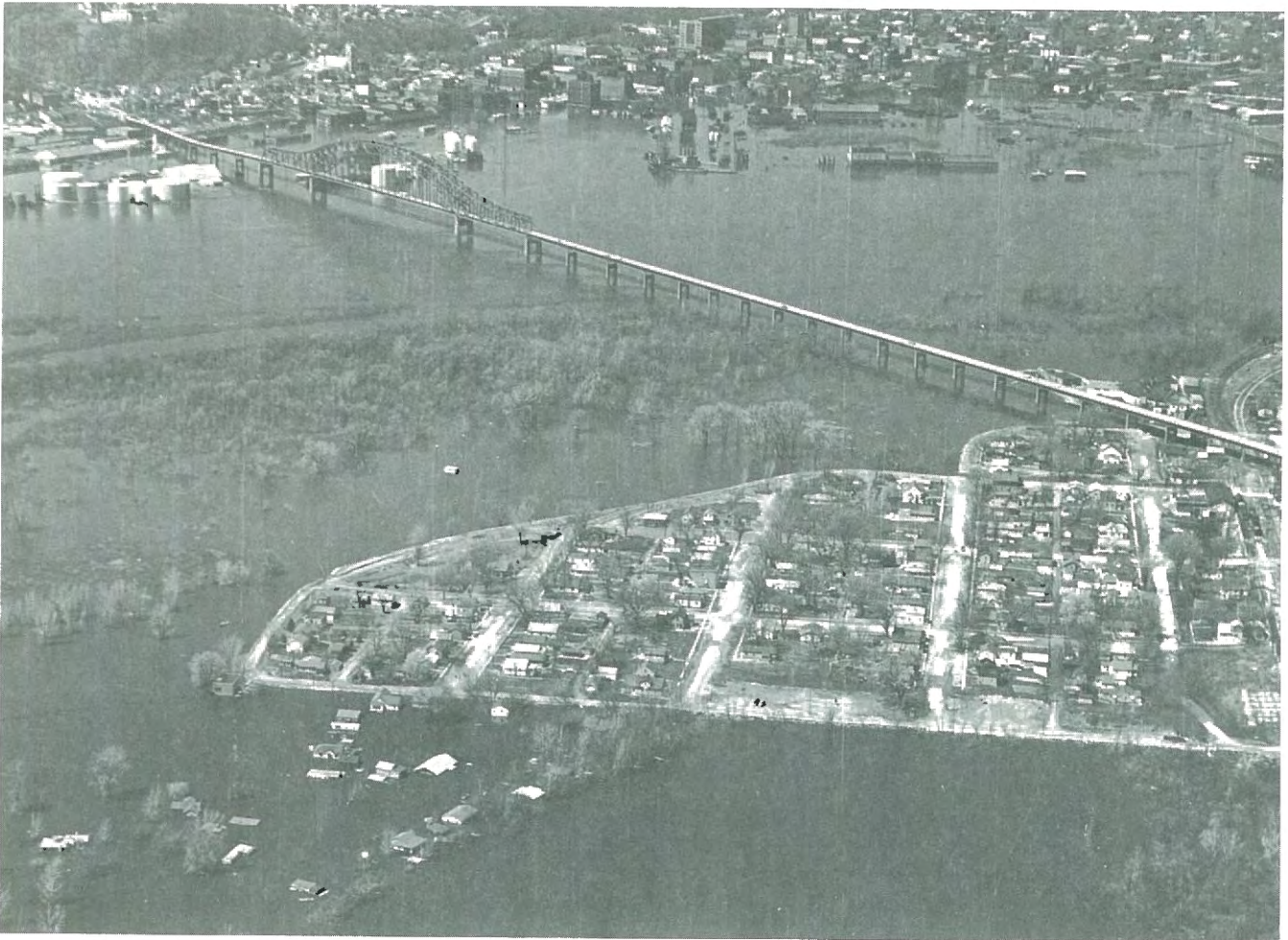
Emergency clay levee in East Dubuque, now a permanent levee system.
